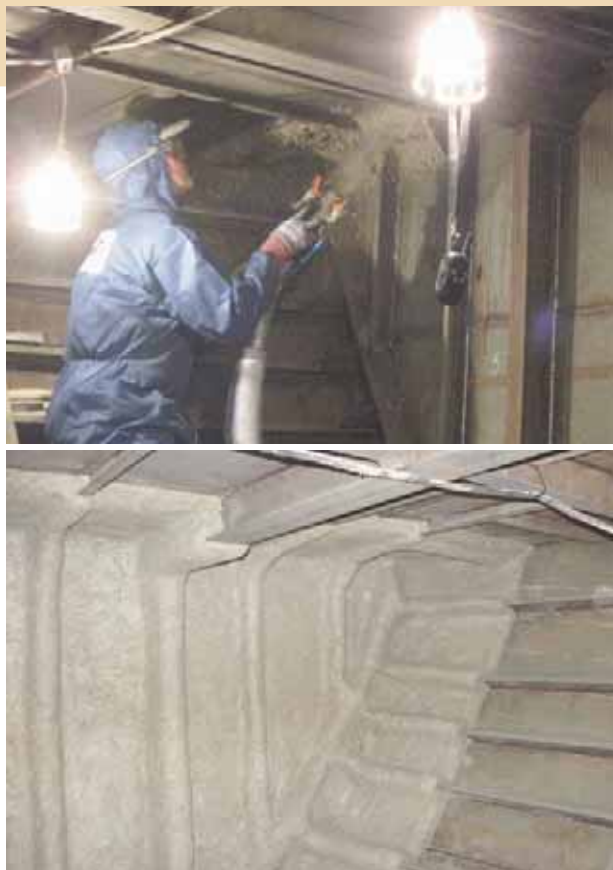
SpreFix®: Isolamento Termico Acustico in classe A60 – applicato a spruzzo SpreFix®: A60 class Thermal Sound Reduction spray-on Insulation
